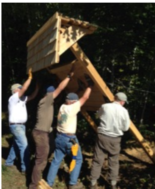
Trail Crew installs a kiosk on the Hills to Sea Trail
