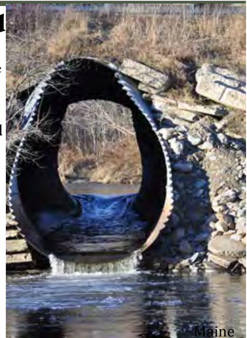
Hung culvert: difficult or impassable
