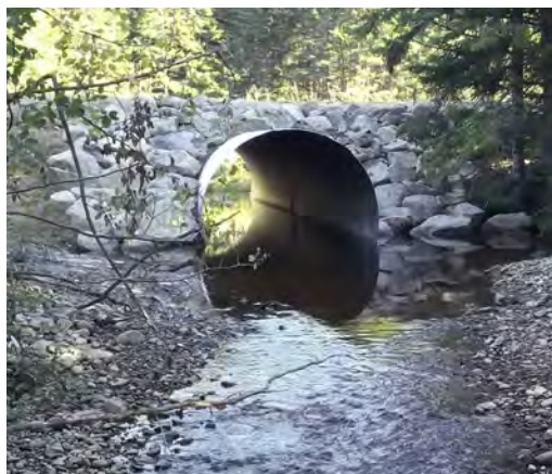
Properly installed culvert with natural bottom, no pour-off. D.O.T. photo
